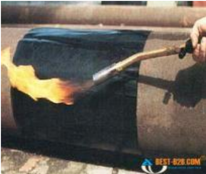
APPLYING A HEAT-SHRINK SLEEVE
