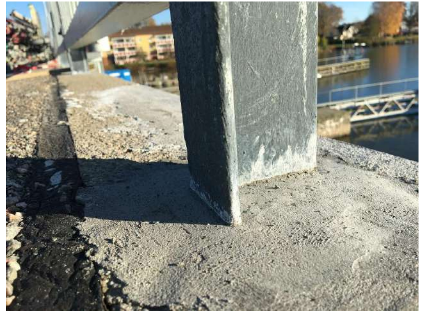
New concrete applied after only one hour
