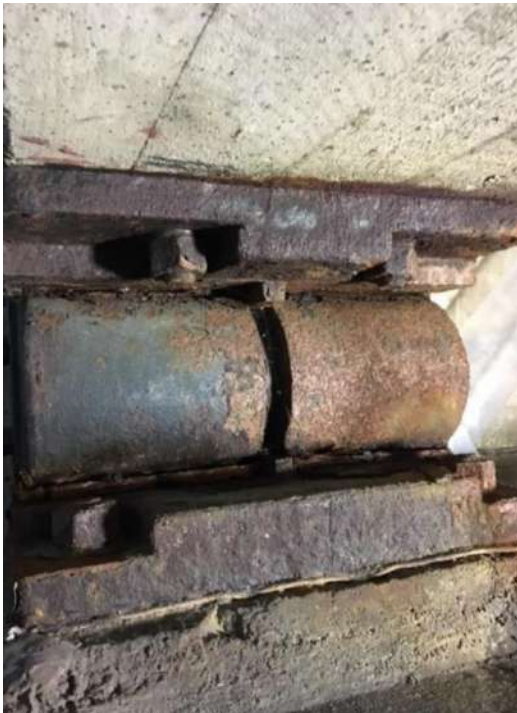
Corroded bridge bearing
