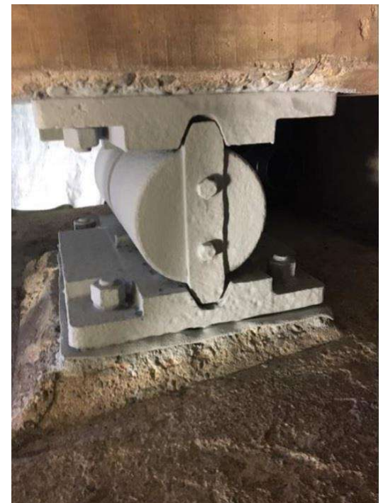
Coated with Zinga 2 x 90 µm
