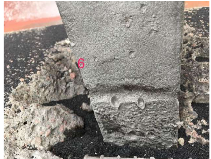
Stanchion base is blast-cleaned
