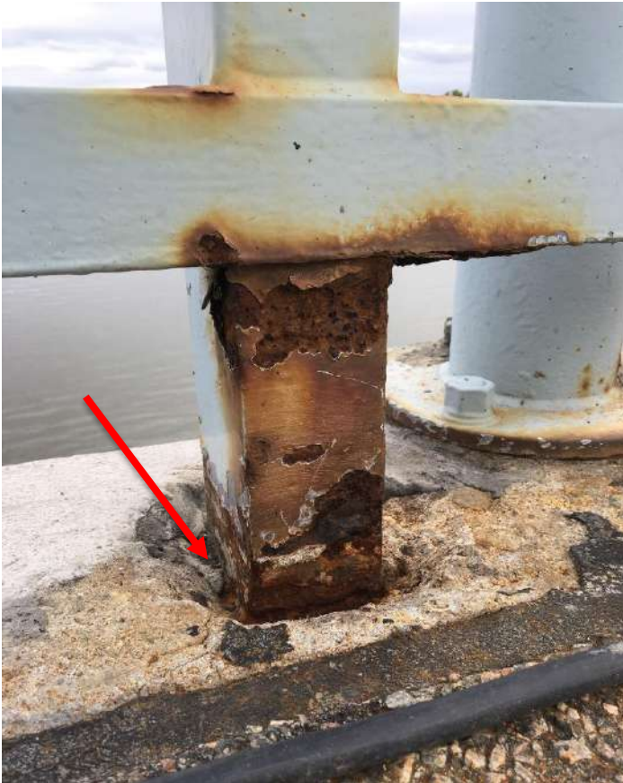
Concrete removed to depth of 70 mm
