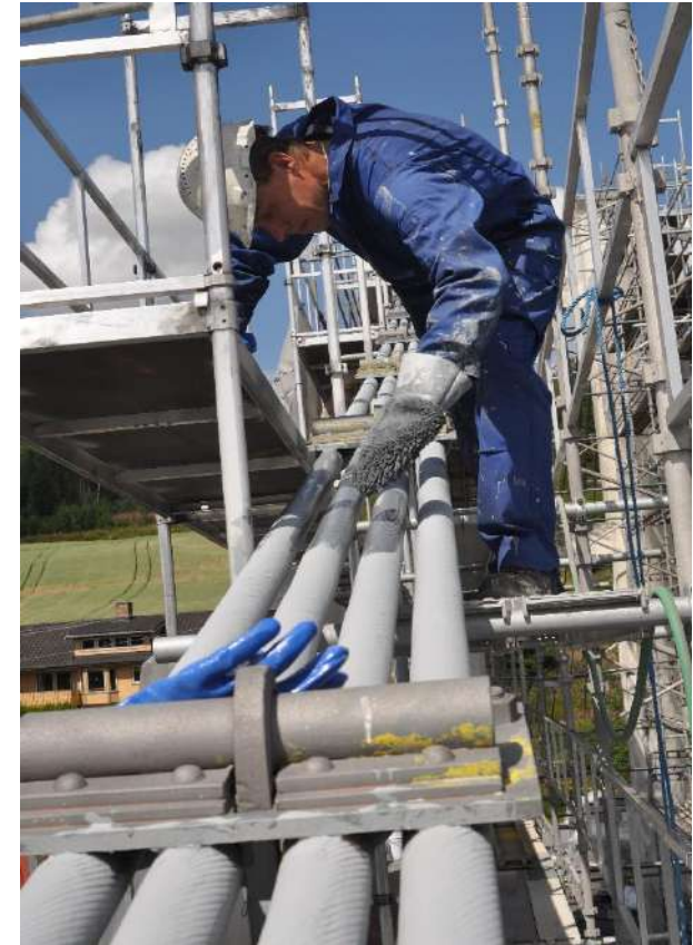
Coating cables using a paint mitt
