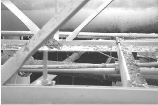
Figure 34. Dust accumulation on roof trusses.
